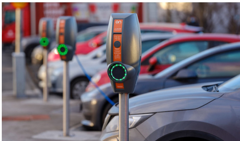
Fig. 4. Bring your own cord EV chargers in Reykjavik, Iceland. Photo courtesy of EV Box.
