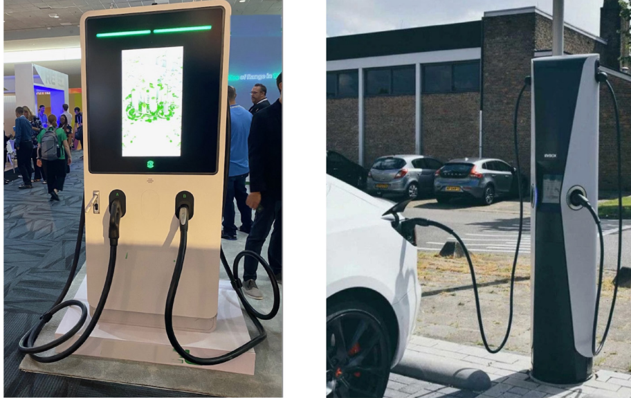
Fig. 3 EV charger cables coiled and lying on the ground at a recent clean energy expo demonstration event, compared with an EV charger deployed in the field equipped with an overhead retractable cable management system.
